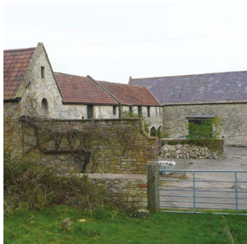
Priory Farm Barns, before and after the conversion and restoration project
